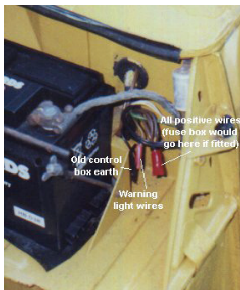
Picture 3: How the wiring looks with no control box.
